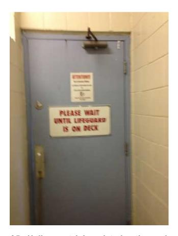
A5 - Hollow metal door deterioration and not barrier free
