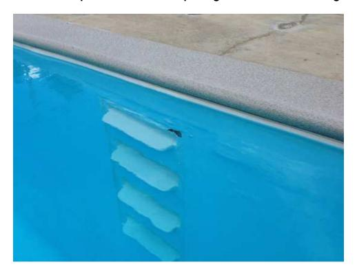
C6 - Liner is damaged and pulling away from concrete
