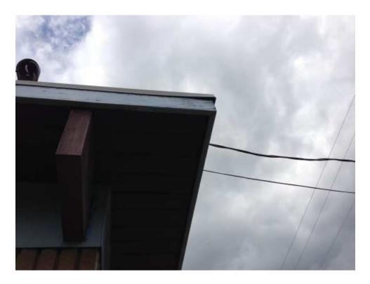
A7 - Painted wood roof fascia requires replacement with metal flashing
