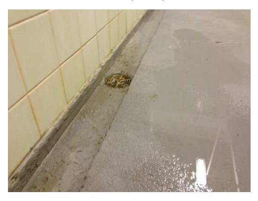
A8- Floor finish has deteriorated and requires replacement
