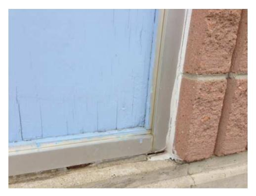
A4 - Caulking and grout filled joints require removal and correction
