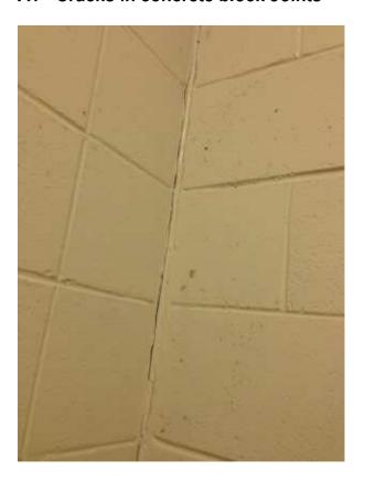
A2 - Cracks in concrete block wall joints
