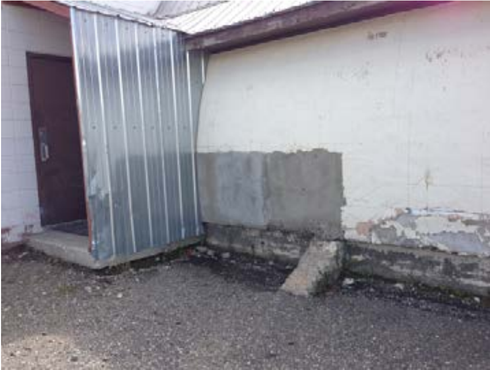
A1 exterior wall and roof envelope requires replacement
