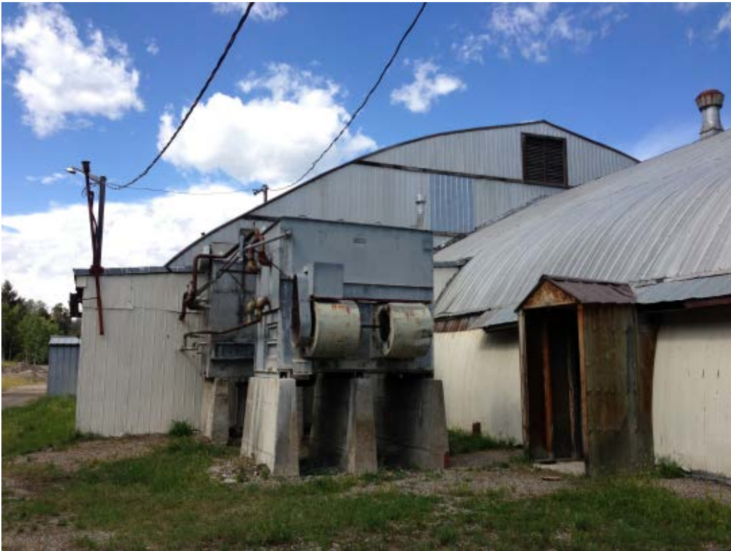
M2 - Original Ice plant system require to be removed.
