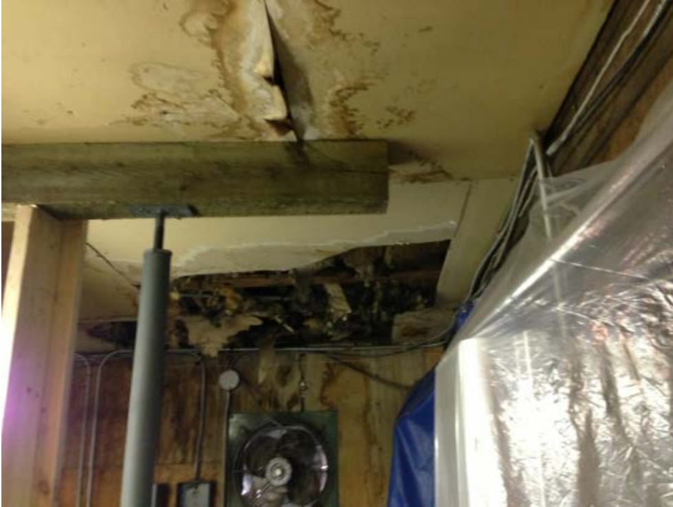
S2 - Shoring of failed roof due to moisture intake and subsequent presences of mould.
