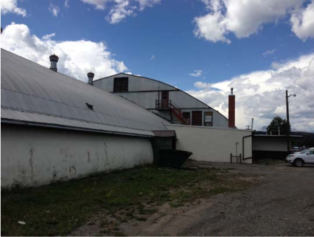
A9 - snow fence and eavestroughing required control water and snow
