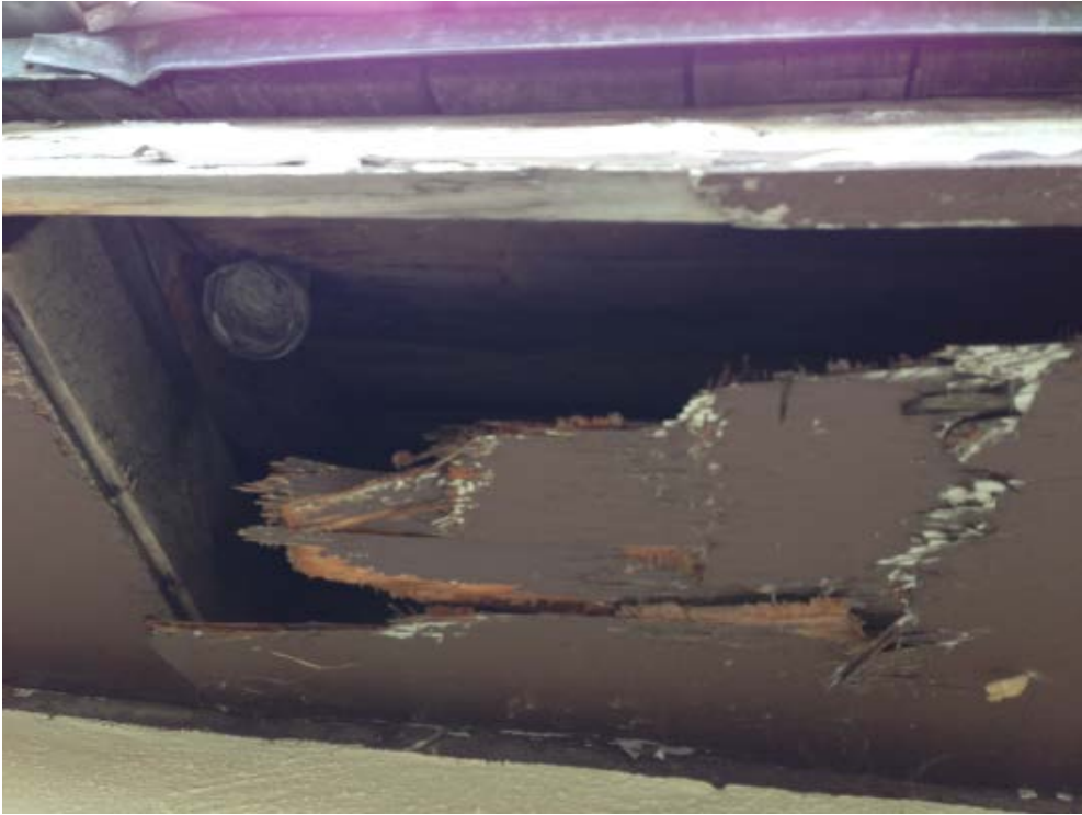
A5- soffit deficiencies
