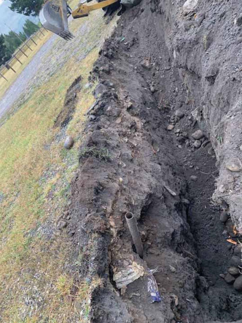
Photograph 43 – Hillcrest Ball Diamond Road – 22HC02, waste (pipe, plastic, metals), burn layer. September 22, 2022.
