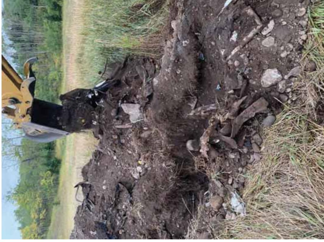
Photograph 41 – Hillcrest Ball Diamond Road – 22HC01, waste (bricks, car parts, plastic). September 22, 2022.
