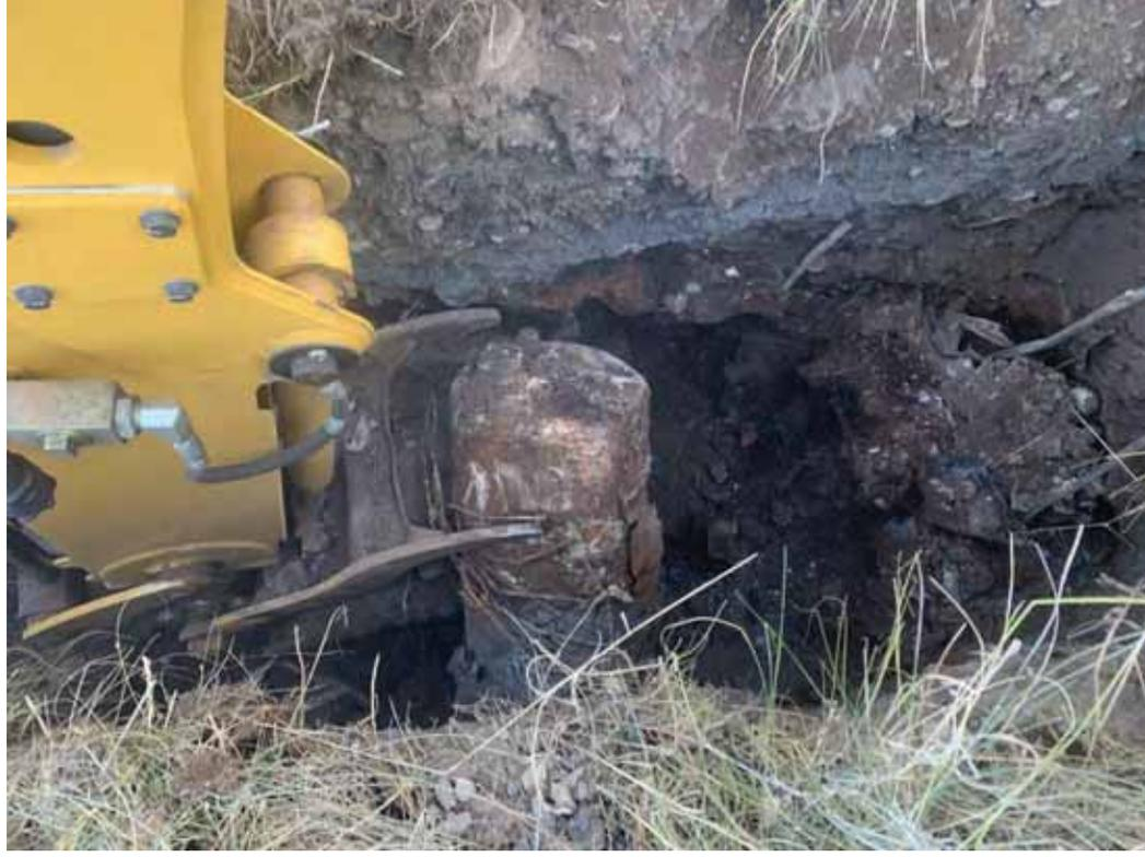
Photograph 27 – Old Sartoris Staging Area – 22OS01 buried tank, burn/ash layer. September 21, 2022.
