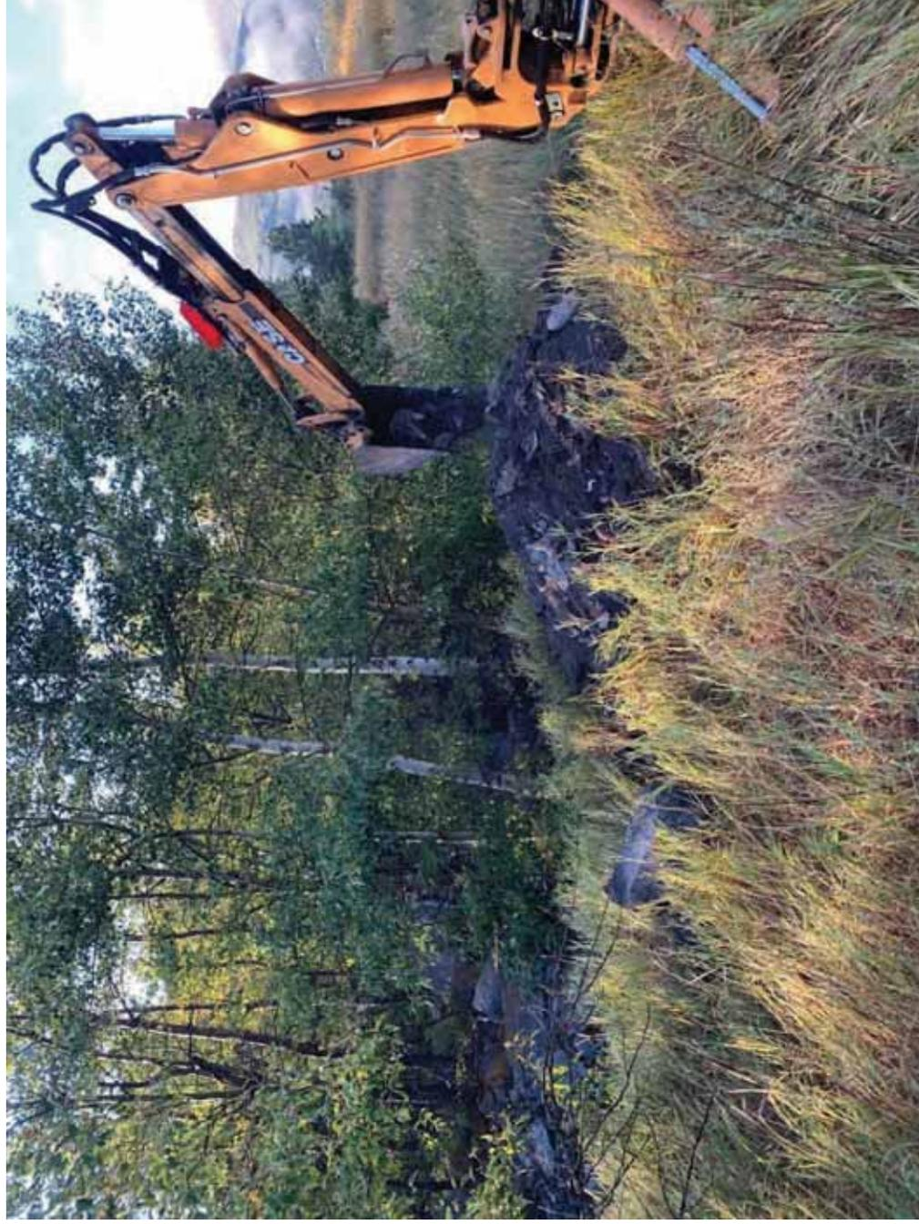
Photograph 64 – Bellevue Old Highway 3 – 22BV02, facing south. Metal waste and boulders excavated from test pit. September 20, 2022.
